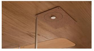
Hold the top magnet firmly in place while aligning with the cardboard magnet template under the surface to find the correct position for the ARC-H. Use a pencil to mark the screw hole locations.
